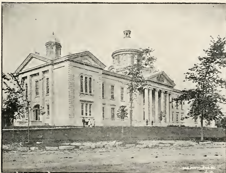
COURT HOUSE, KINGSTON, ONT.
